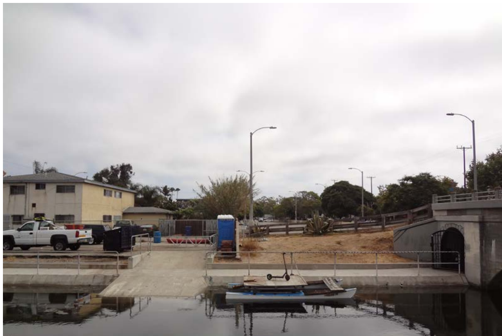
Photograph 4: View of the Project site facing approximately northeast depicting the onsite portion of the Grand Canal in the foreground, prostrate knotweed provisional herbaceous alliance in the middleground, and disturbed/developed land use in the background.
