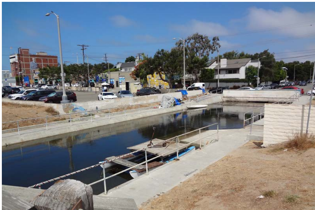
Photograph 6: View of the Project site facing approximately west depicting the onsite portion of the Grana Canal with prostrate knotweed provisional herbaceous alliance visible in the foreground and background.
