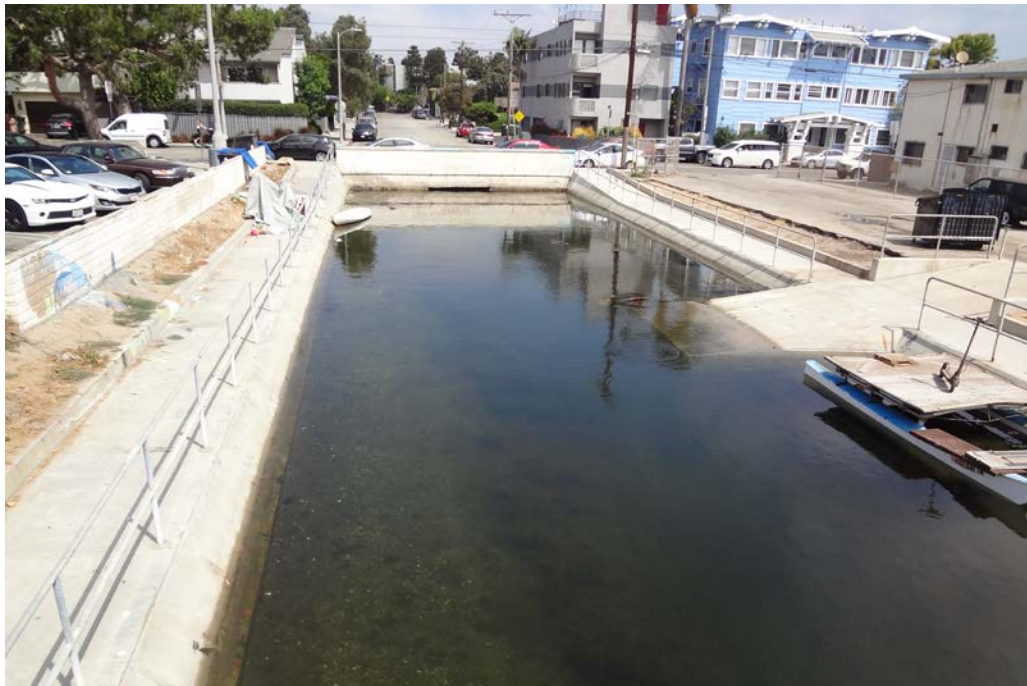
Photograph 5: View of the Project site facing approximately northwest depicting the onsite portion of the Grana Canal. Note the presence of water staining along the concrete walls of the Canal.
